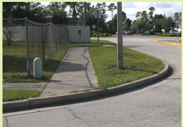
Sidewalks do not include curb ramps on Cedar Highlands Boulevard
