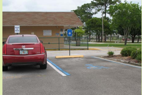
The accessible parking stall on the south side of the school needs a connecting crosswalk to the curb ramp
